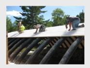
The FRP tubes are the only formwork required, saving labor, time, and money.
